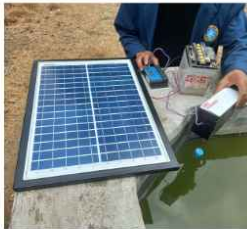
Gambar 5. Alat Monitoring Water Turbidity Berbasis PLTS
