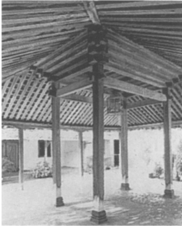
Figures 3: The four master pillars of an ideal Javanese mosque. Source: (Kusno, 2003)
